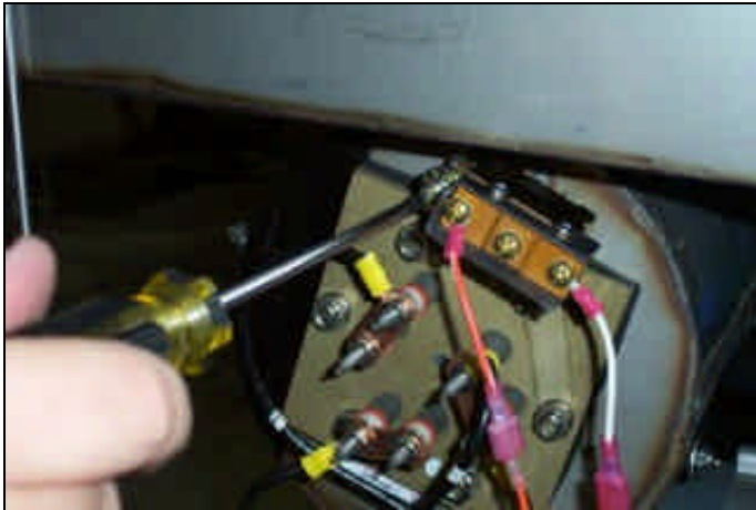
Calibrating the new thermostat.
